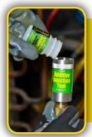
Easily Injected into an Operating System with ½ oz QwikInjector® (P/N QT2510)
