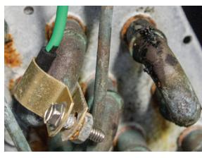
Installing temperature sensor of the QwikSwap® on the coil
