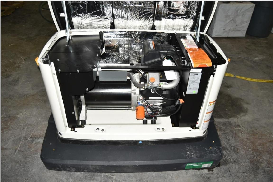
**Figure D-4. Generator Bolted to the *QwikHurricane*<sup>®</sup> Generator Pad<sup>™</sup>.**
