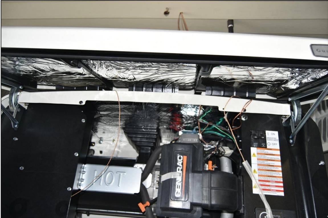
**Figure D-7. View of Spark Igniter and Leak Tube for Tests 1 and 2.**
