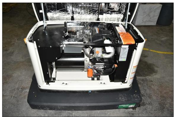
Figure D-4. Generator Bolted to the  $QwikHurricane^{\otimes}$  Generator Pad<sup>TM</sup>.
