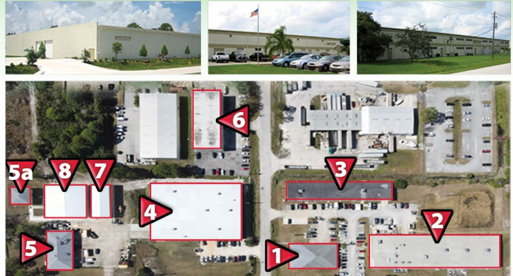
1 - ENGINEERING OFFICES 4 - PRODUCTION 6 - CONTROLLED-ATMOSPHERE BRAZING FACILITY 2 - RESEARCH & DEVELOPMENT 5 - PRODUCT DEVELOPMENT 7 - SHEET METAL FABRICATION 3 - RESEARCH & DEVELOPMENT 5a - MAINSTREAM EBEAM 8 - ROTOMOLD PRODUCTION
